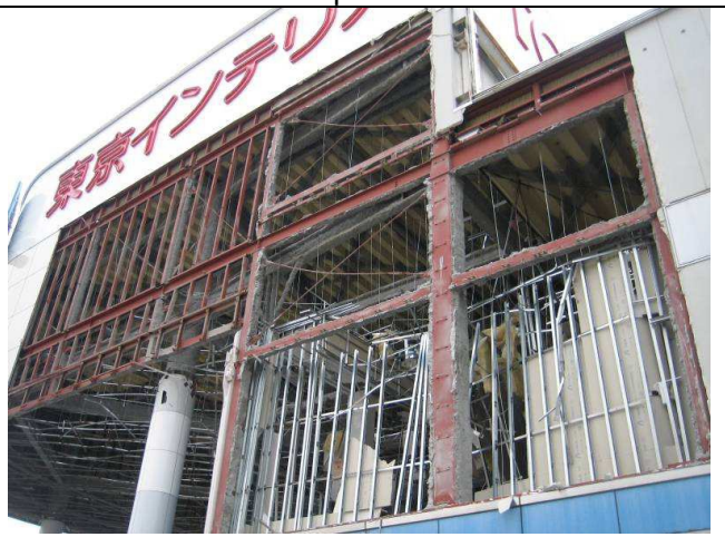
Photo 4: Fall of exterior curtain walls
