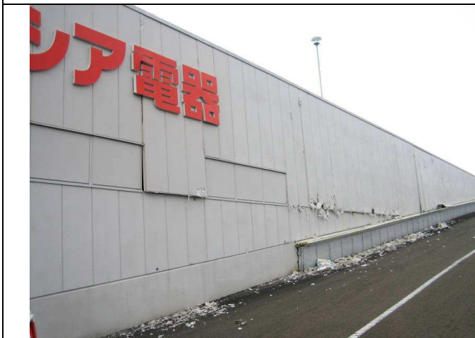
Photo 4: Breakage of ALC (autoclaved light-weight concrete) panel (Building 2)
