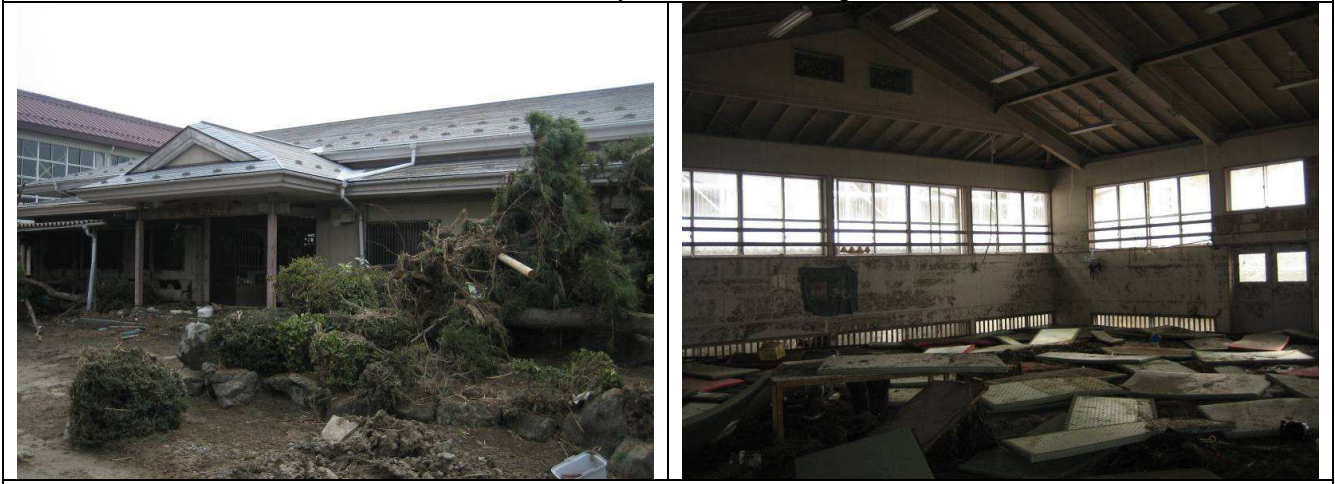
Photo 10: Gymnasium for military arts (No lighting fixture fell)
