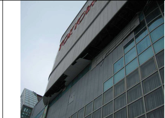
Photo 2: Fall of ceiling (Building 1)
