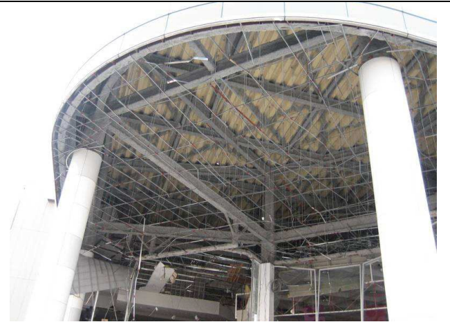
Photo 2: The ceiling dropped and roof skeleton is exposed
