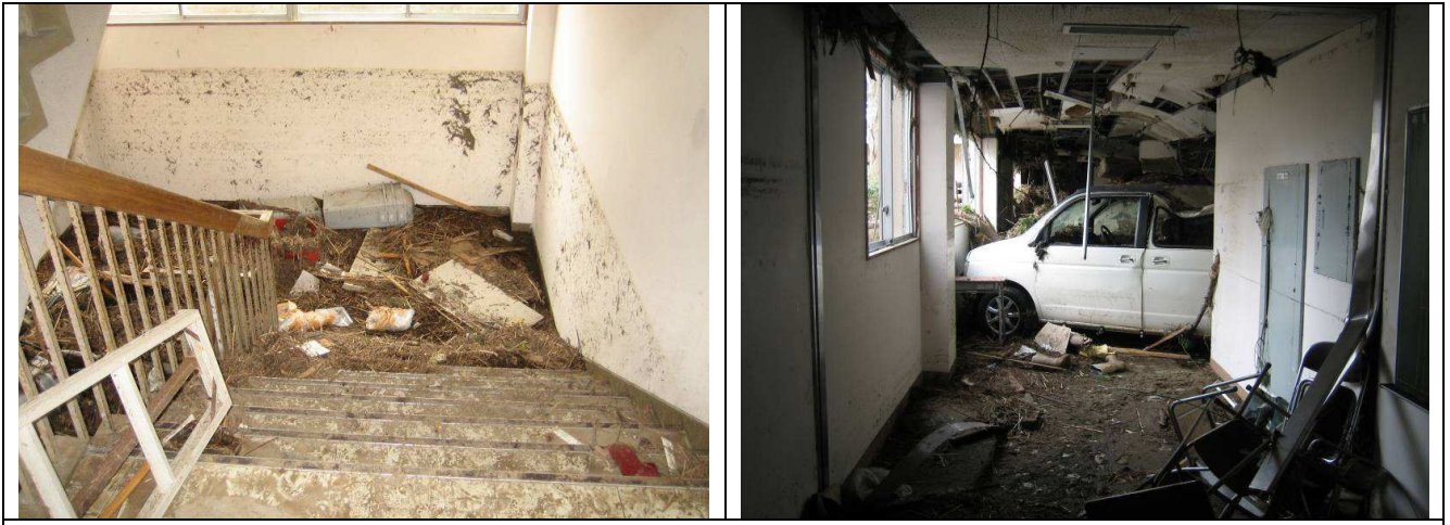
Photo 8: Inside of the Central Building
