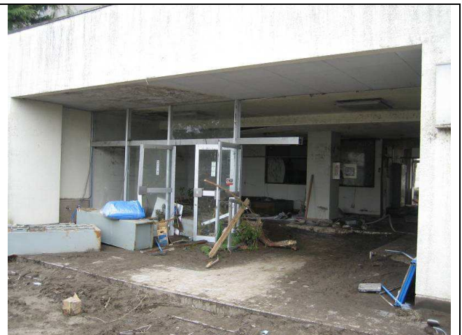
Photo 2: Entrance damaged by the tsunami
