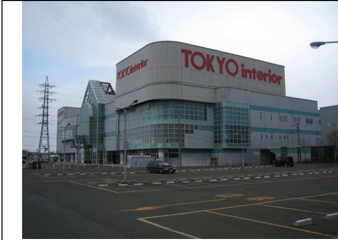
Photo 1: Exterior overall view of Building 1
