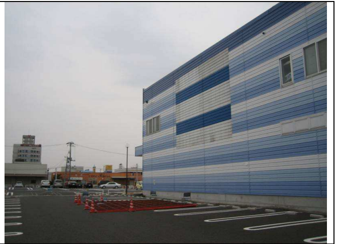
Photo 12: Fall of exterior panel to parking lot
