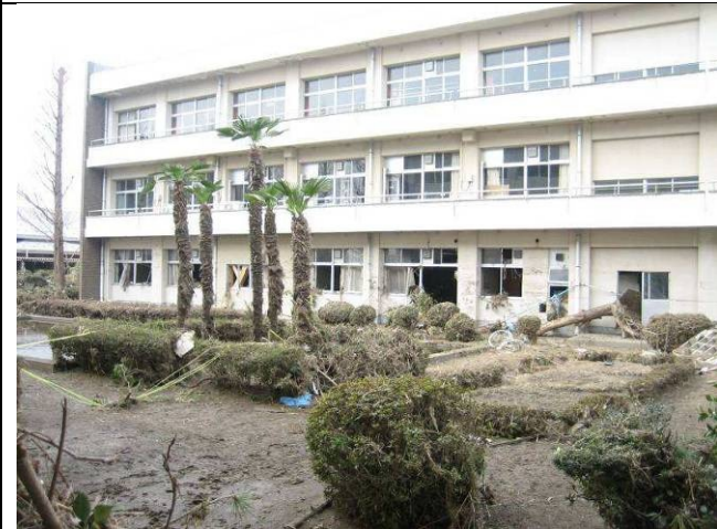
Photo 5: South face of the North Building
