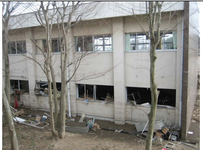
Photo 6: North face of the North Building
