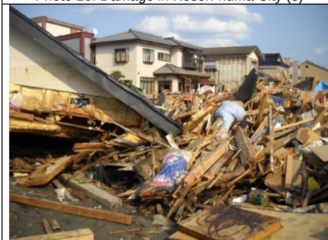
Photo 22: Damage in Kesen-numa City (5)
