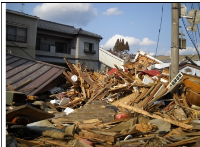
Photo 20: Damage in Kesen-numa City (3)
