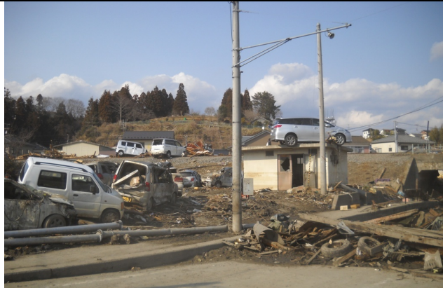
Photo 15: Tsunami crossed the railway.
