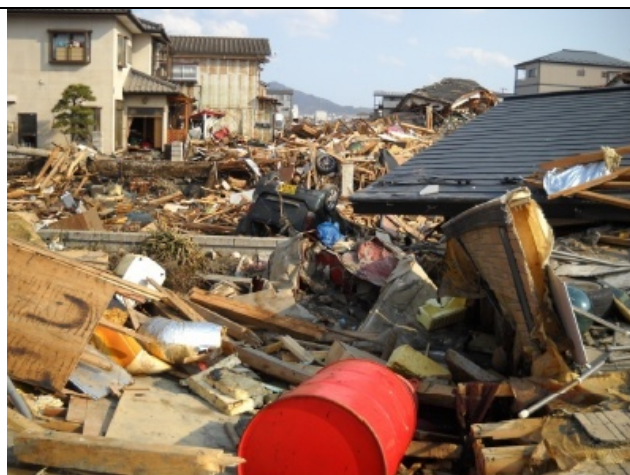
Photo 21: Damage in Kesen-numa City (4)
