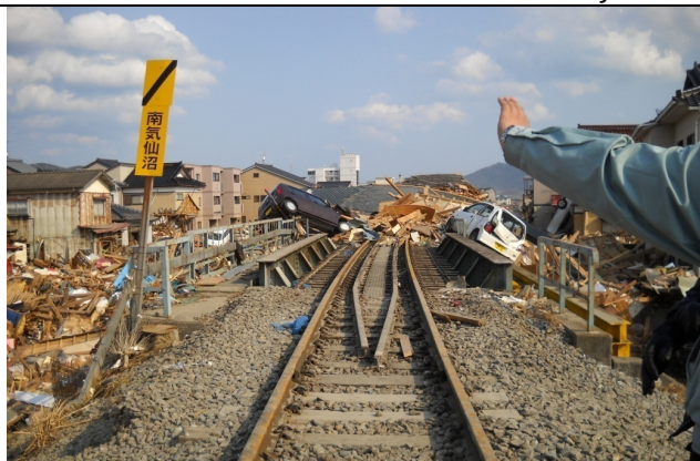
Photo 17: Rubbish was brought across the railway.
