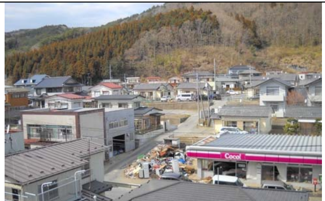
Photo 7: Onagawa High School is located on a hill.
