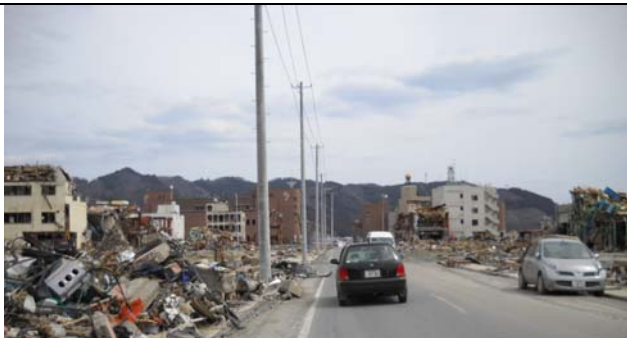
Photo 29: Reinforced concrete and steel structures remained standing near the port.
