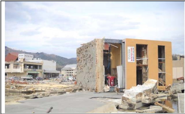
Photo 41: Overturned RC buildings (1).
