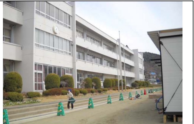
Photo 2: No damage in the school building.
