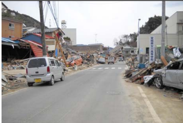
Photo 17: Some houses were standing and others collapsed in Zone B.
