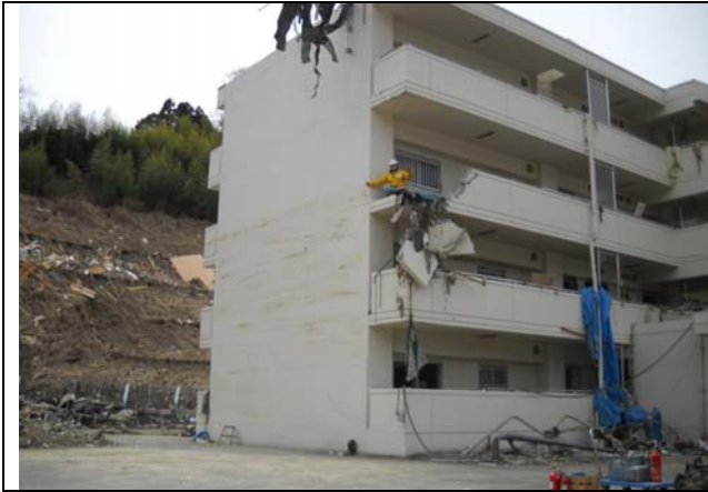
Photo 38: A four-story RC condominium.
