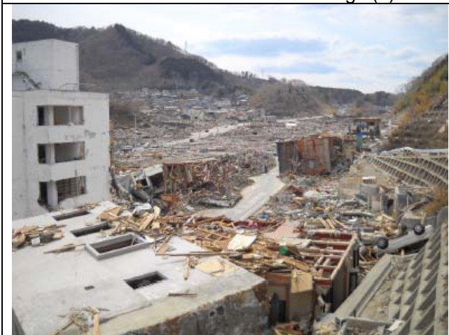
Photo 43: Overturned RC buildings (3).
