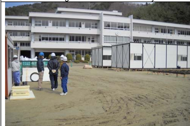
Photo 3: Temporary houses were under construction on the play ground.
