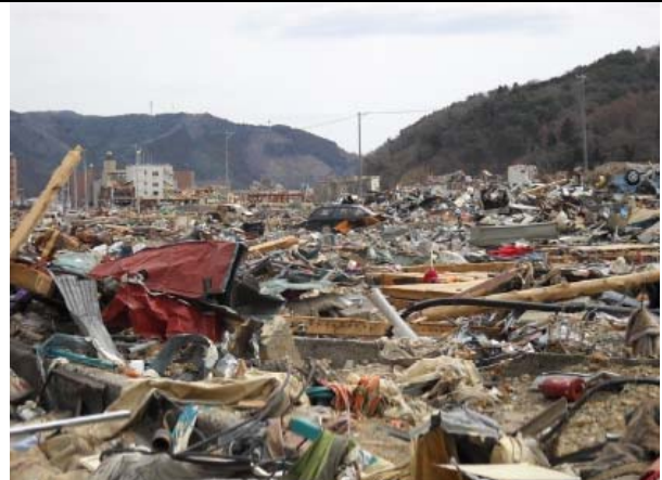
Photo 28: Totally destroyed houses in Zone C (4)
