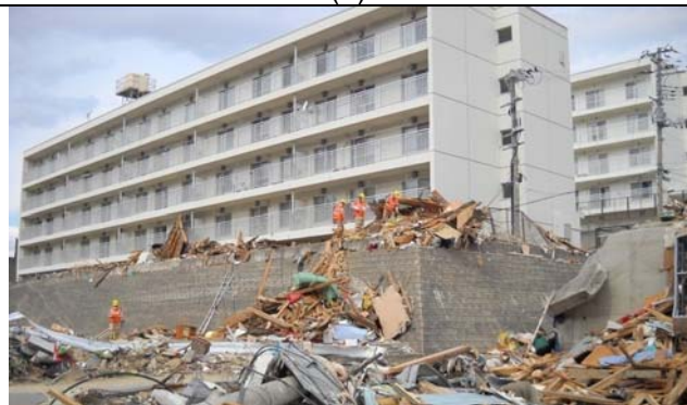
Photo 24: Undamaged reinforced concrete condominium buildings on slightly higher altitude
