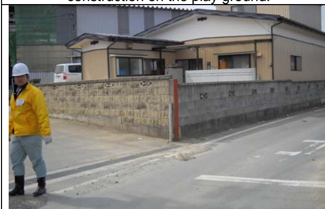
Photo 5: Houses protected by concrete walls suffered no damage.
