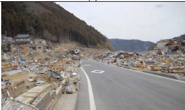
Photo 23: Total destruction of houses in low land (3).
