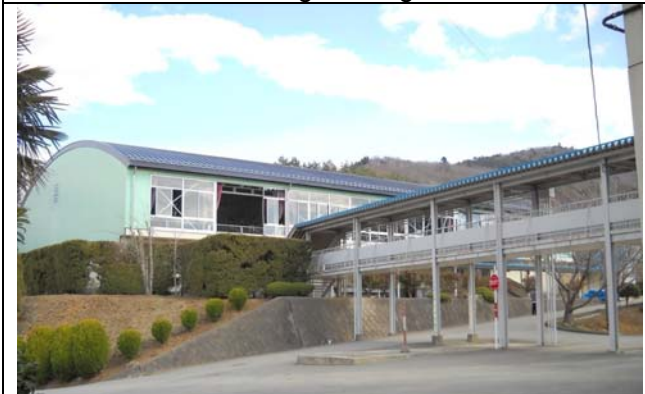
Photo 8: Window glasses were broken in the gymnasium (1).
