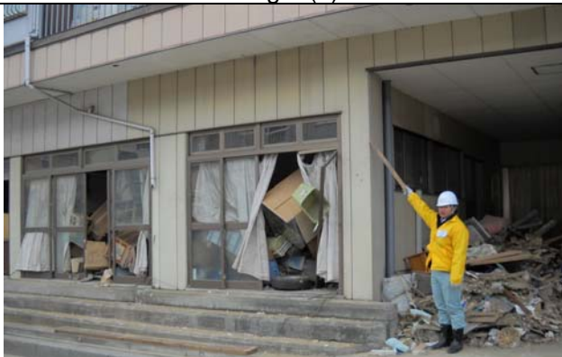
Photo 14: Damage became significant as the tsunami height reached approx. 1.8 m.
