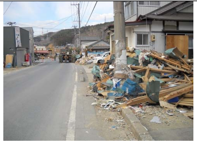
Photo 13: Damage increased with descending height (2)
