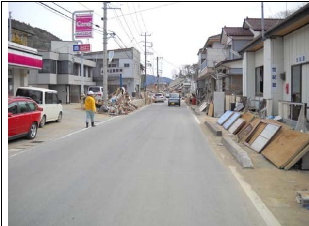
Photo 12: Damage increased with descending height (1)
