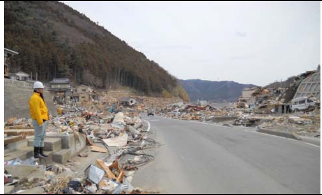
Photo 22: Total destruction of houses in low land (2).
