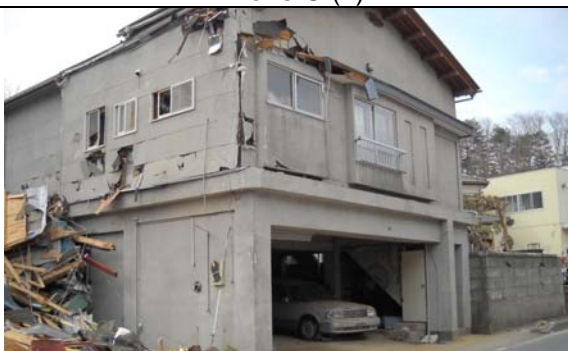
Photo 20: First story RC and second story timber house in Zone C.
