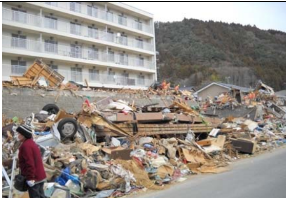
Photo 18: Most timber houses were washed away in Zone C (1).
