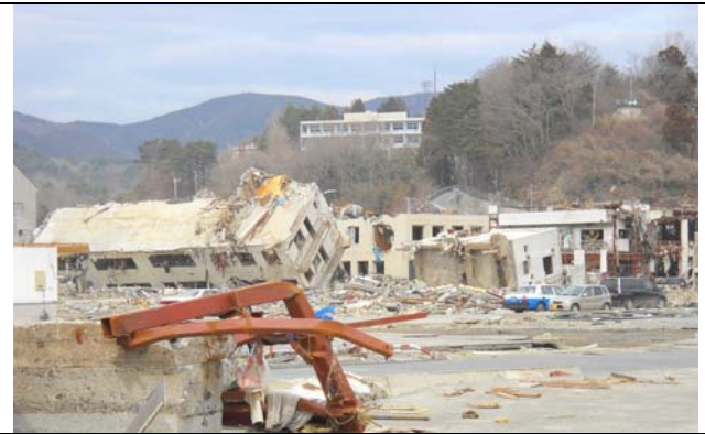
Photo 42: Overturned RC buildings (2).
