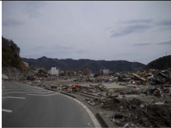
Photo 27: Totally destroyed houses in Zone C (3)
