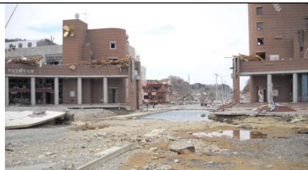
Photo 31: The corridor between the two buildings was washed away.
