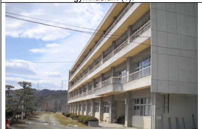
Photo 10: The school building suffered no damage.
