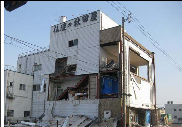
Photo 15: Fall of external non-structural walls from a three-story steel commercial building
