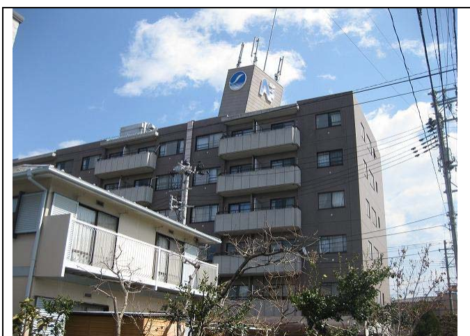
Photo 5: A tilted penthouse of a six-story reinforced concrete condominium building
