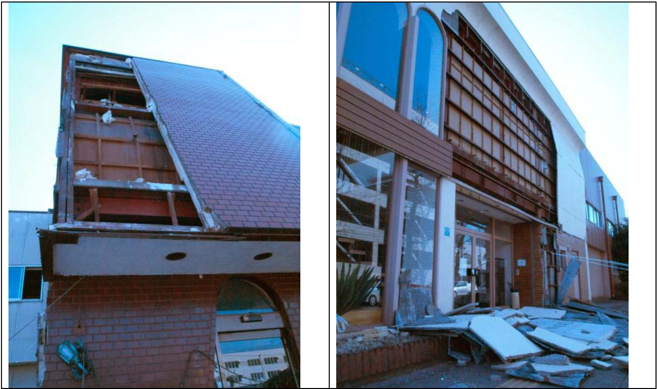
Photo 14: Fall of exterior curtain walls in steel construction
