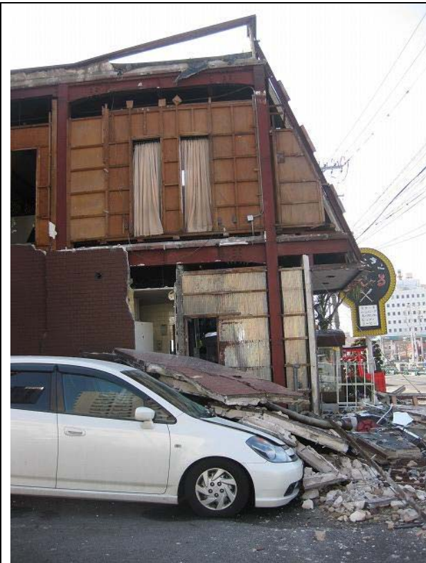
Photo 9: Exterior finishing fell from a two-story steel building
