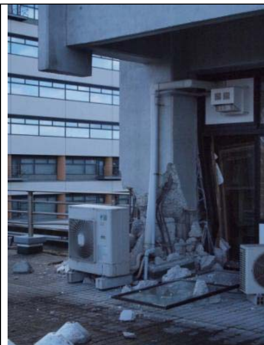
Photo 3: Damage of north-east corner column
