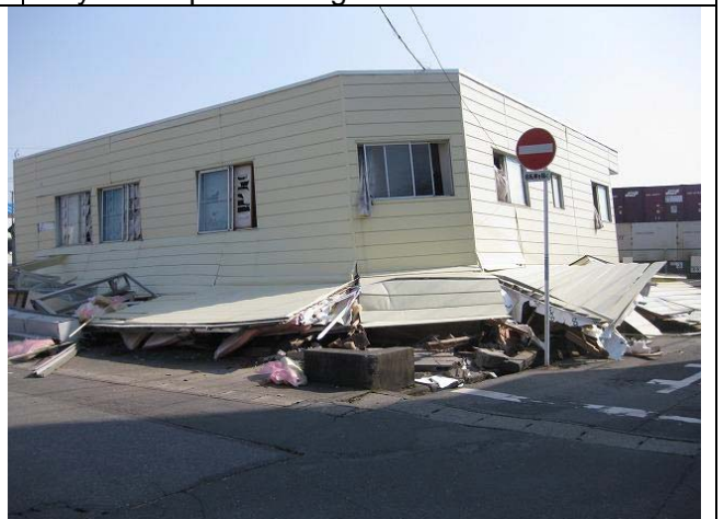
Photo 9: Collapse of a two-story house for combined use for shop and residence
