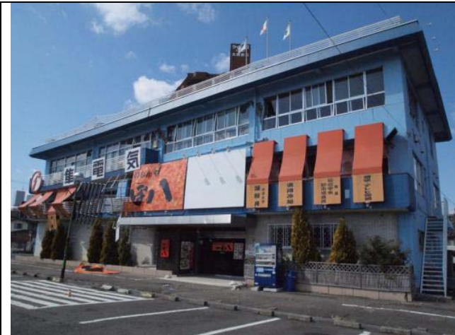
Photo 6: Collapse in the second story of a three-story reinforced concrete building in Yamato-machi 5-chome.
