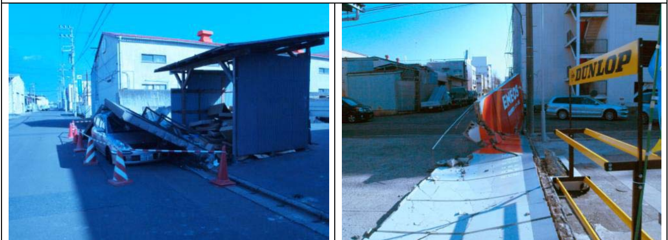
Photo 15: Overturned concrete block fences in Oroshi-machi, Wakabayashi-ku
