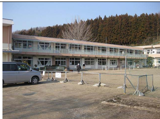
Photo 14: Overview of Uenome Elementary School (No damage)
