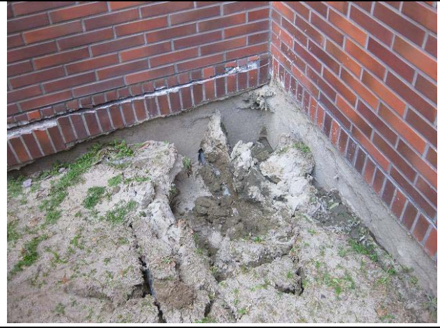
Photo 11: Boundary of foundation and ground at the base of the 11-story reinforced concrete hotel building
