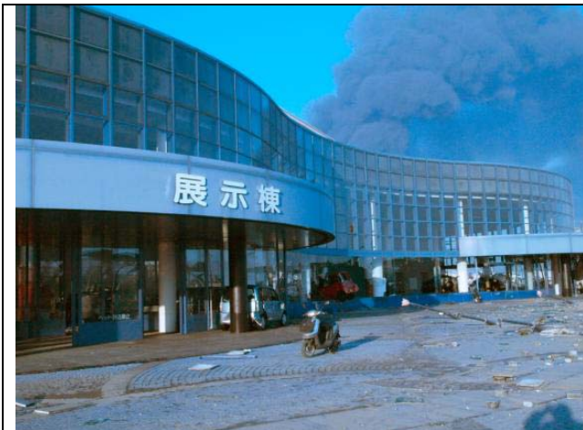
Photo 22: Damage of Miyagi Yume Messe by tsunami
