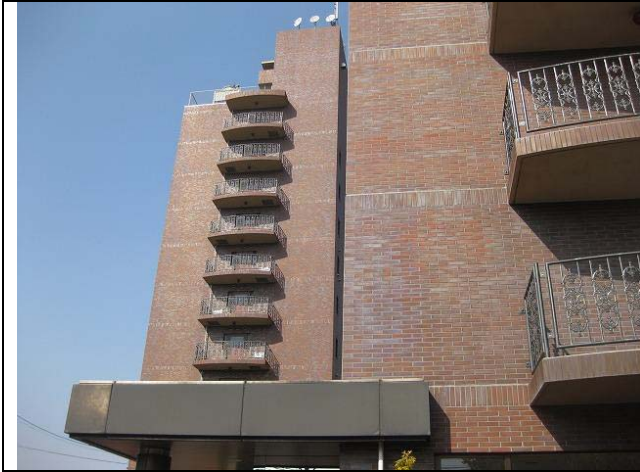
Photo 10: Tilting of a 11-story reinforced concrete hotel building
