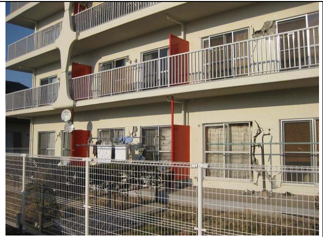
Photo 17: Shear failure of non-structural exterior walls
