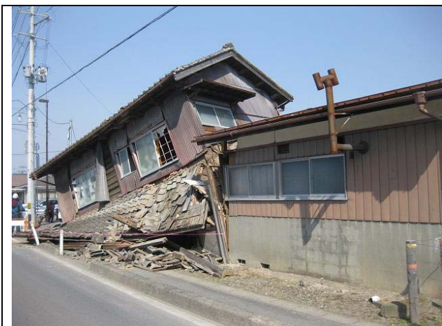
Photo 2: Collapse of a two-story timber house
