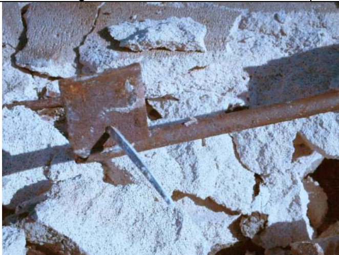
Photo 11: Detail of fastener (anchor) of fallen ALC exterior wall
