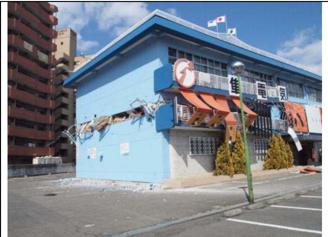
Photo 7: Collapse in the second story
