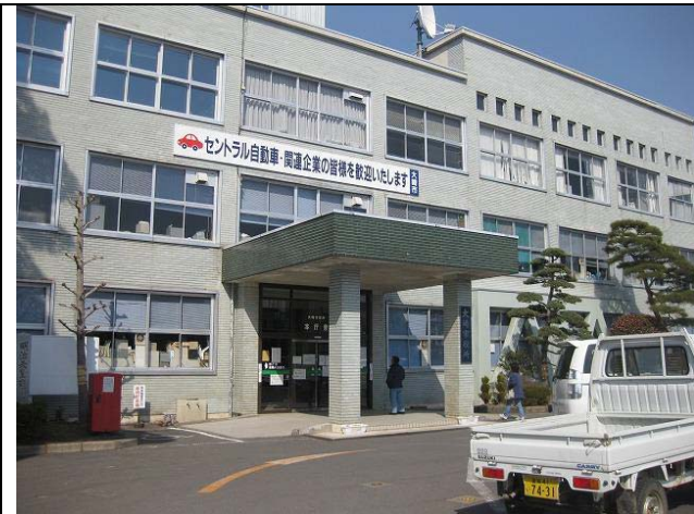
Photo 4: Ohsaki City Municipal Building
