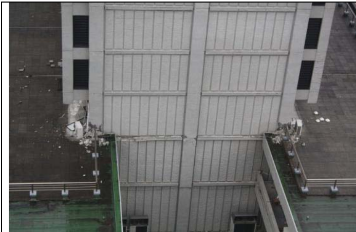
Photo 1: Damage of end walls from roof of the adjacent building
